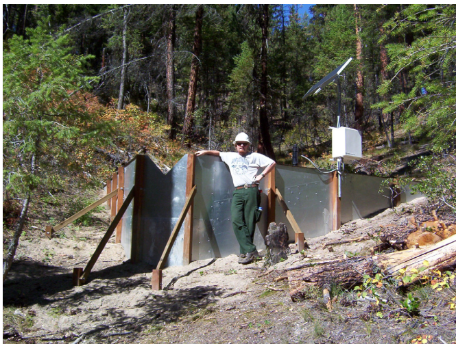
Figure 5. V-notch weir and headwall on one of the watersheds destined for a wildfire treatment in the Boise Basin Experimental Forest.
